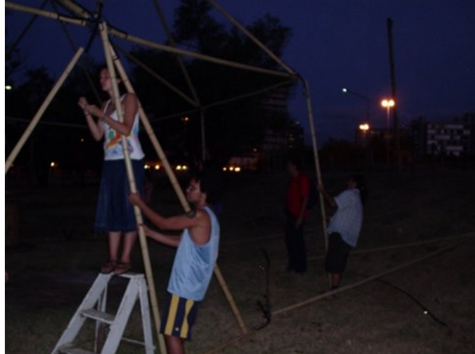
Construction of Geodesic structure
