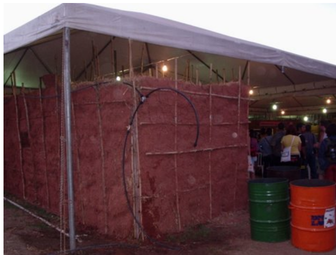
Health center: the wall was built with adobe
